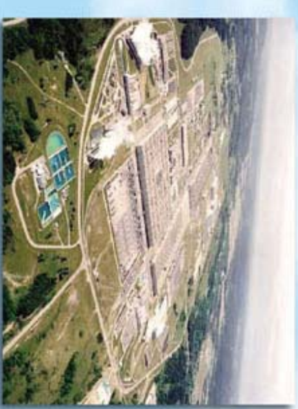
The Portsmouth Gaseous Diffusion Plant began removing the first of 16 inactive facilities in February of 2006.
