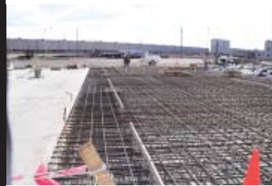
Conversion Building Foundation
