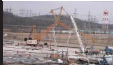
Utilities Installation and Foundation Work
