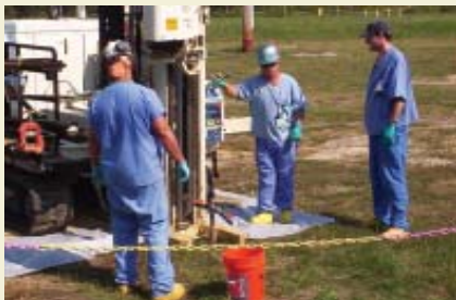
Initial Results Positive on Oxidant Treatment of Groundwater, page 3
