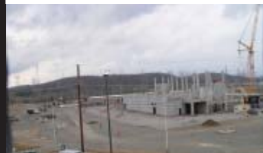
Conversion Building, Late March 2006
