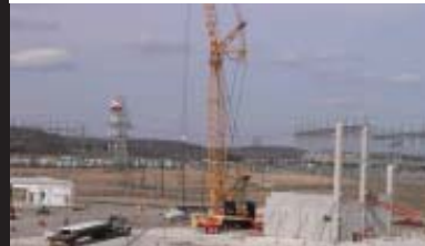
Initial Conversion Building Construction
