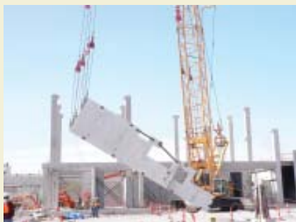
Work Progresses on DUF6 Conversion Plant, page 2
