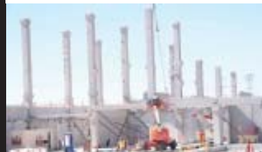
Work Progresses On Conversion Plant
