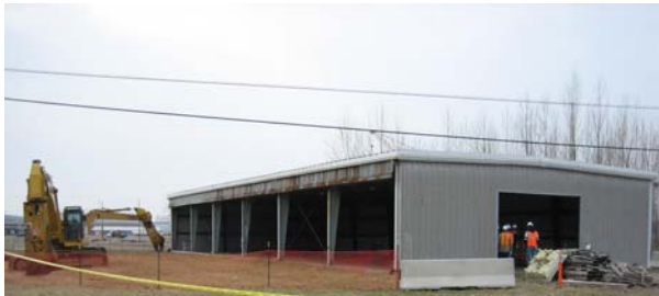
X-740 Waste Oil Storage Facility before demolition
