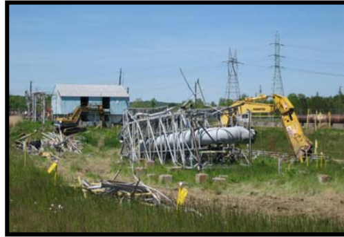
Pictured above is the X-344E stack after dismantlement.
