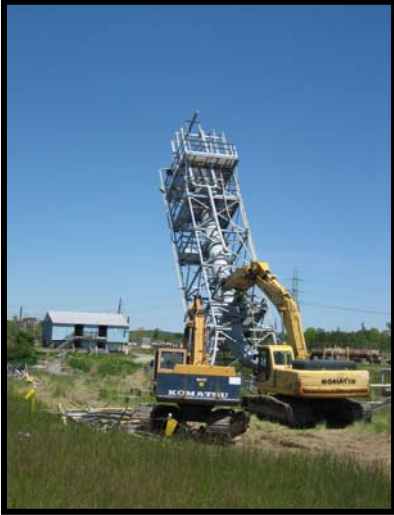
X-344E Gas Ventilation Stack Being Dismantled on May 23, 2006.
